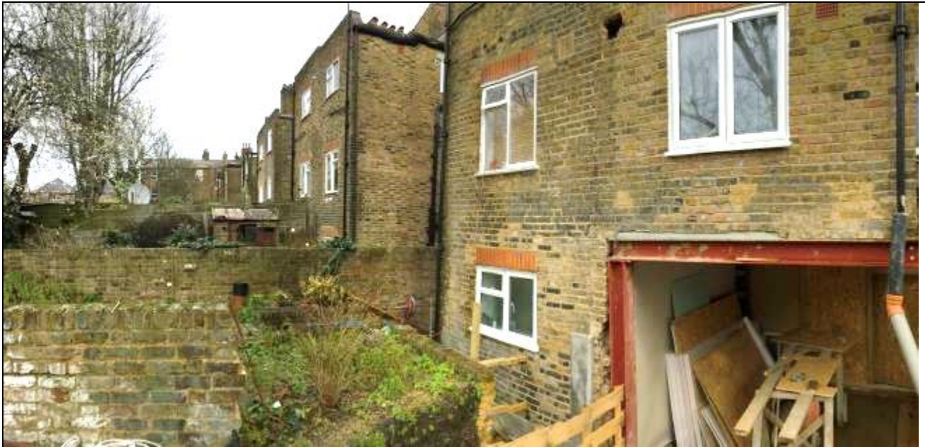
View North and boundary with No 62
